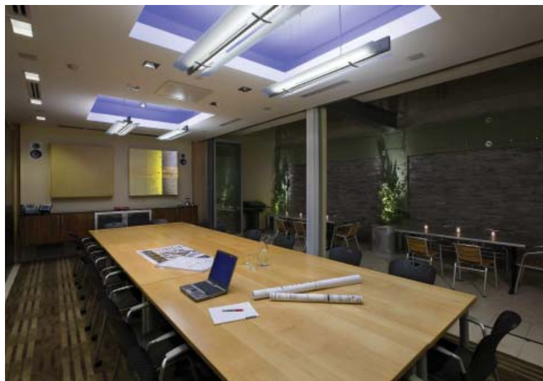
LEFT: color changing LED cove lights, direct/indirect fluorescent pendants, MR-16 downlights and compact fluorescent wall washers all dim separately providing the conference room with multi-scene presets. Interactive touch screen operates A/V equipment and drapes providing users with one-touch scenes for any occasion.
